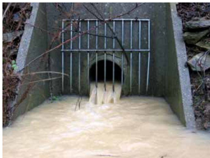
Figure 9: Subsurface drainage outlets
